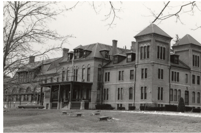
Westborough State Hospital c. 1975 Photo courtesy of Westborough Center for History and Culture.
